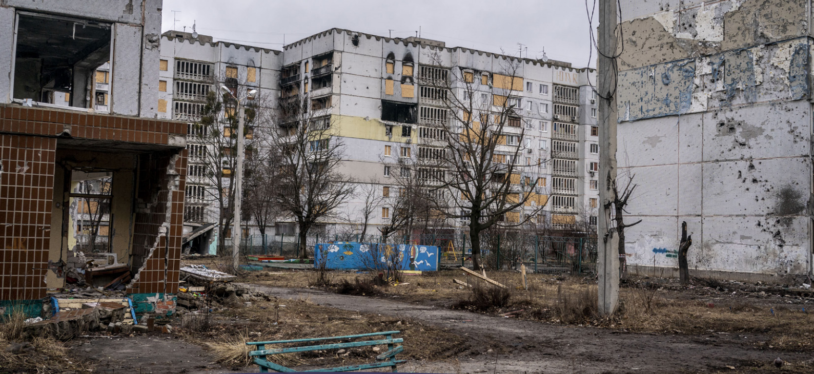
Damaged buildings in Kharkiv, March 2023. © Jose Colon/Anadolu Agency via Getty Images
